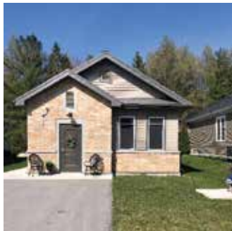
Milne pumphouse (PH) Well 4
