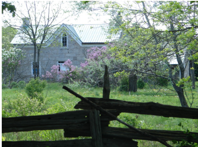
Photo 17 – 1 ½ storey stone farmhouse at 4958 sixth Line
