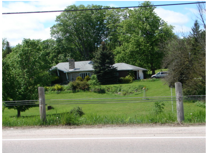
Photo 14 – Mid-twentieth century bungalow off-site on south east severance (8540 Hwy. 7)
