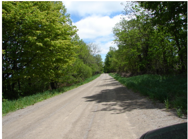
Photo 3 – Sixth Line looking south
