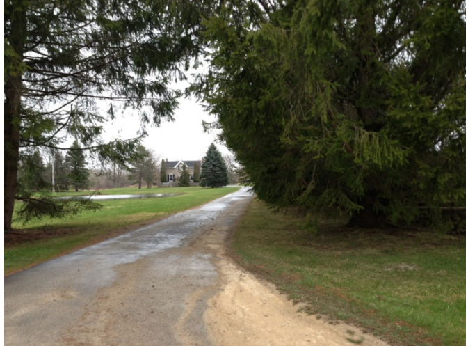
Photo 16 – 1 ½ storey stone farmhouse at 4963 Sixth Line
