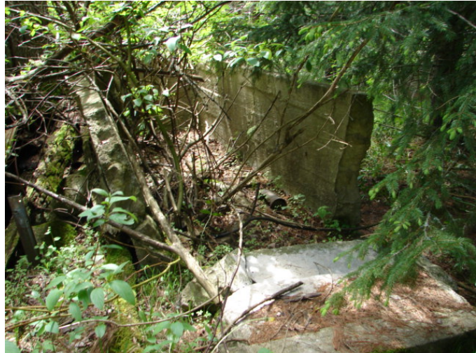
Photo 7 – Concrete cistern at farmhouse site
