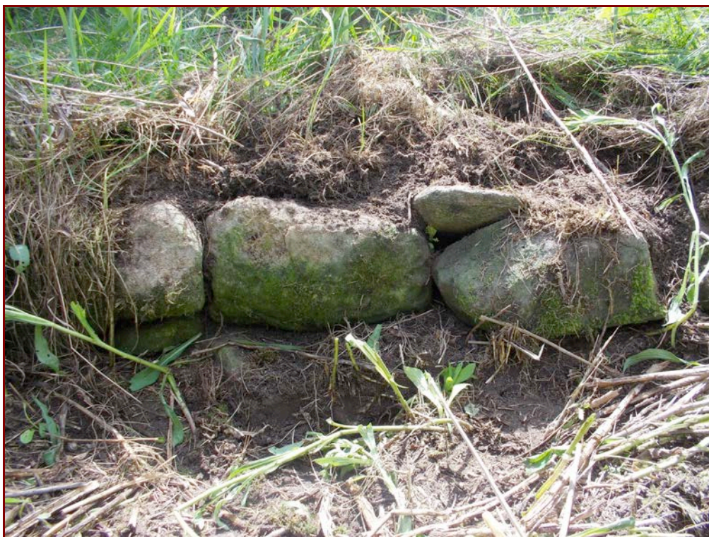
IMAGE 19 FOUNDATION WALL TAKEN FROM INSIDE FOUNDATION
