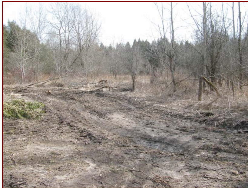
IMAGE 6 SKIDDER PATH ALONG WESTERN EDGE OF THE STREAM LOOKING TO THE NORTHEAST.
