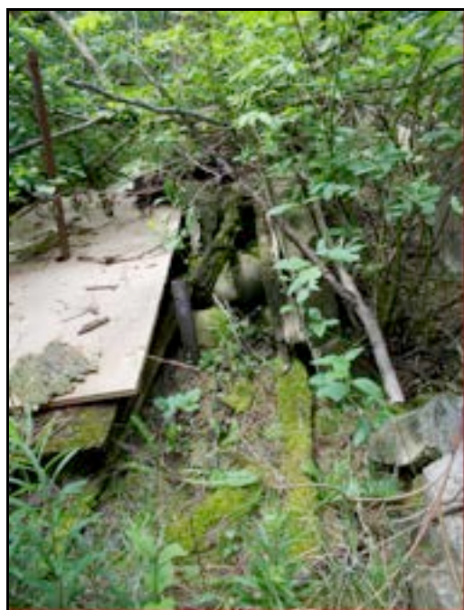
IMAGE 18 WELL, AREA JUST SOUTH OF CONCRETE BOX
