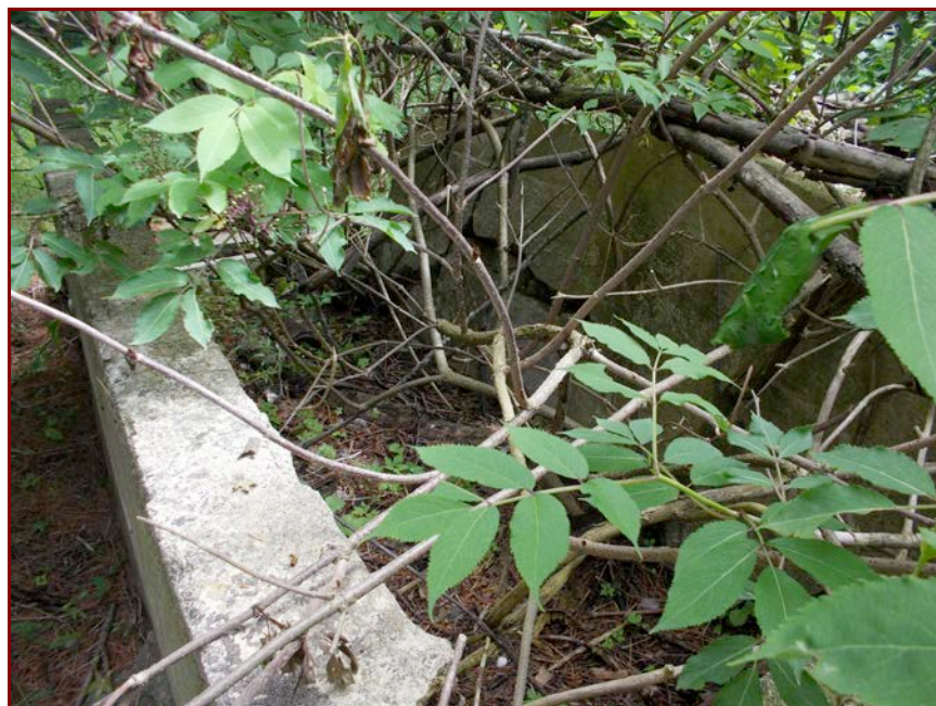
IMAGE 17 INTERNAL VIEW OF CONCRETE BOX
