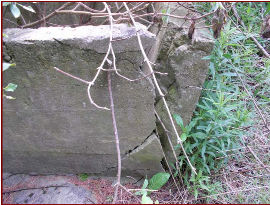
IMAGE 16 CONCRETE BOX LOCATED NORTH OF THE WELL
