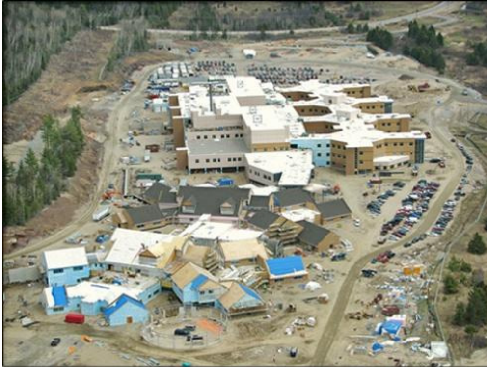
Figure 2-18 North Bay Regional Health Center (Under Construction)
