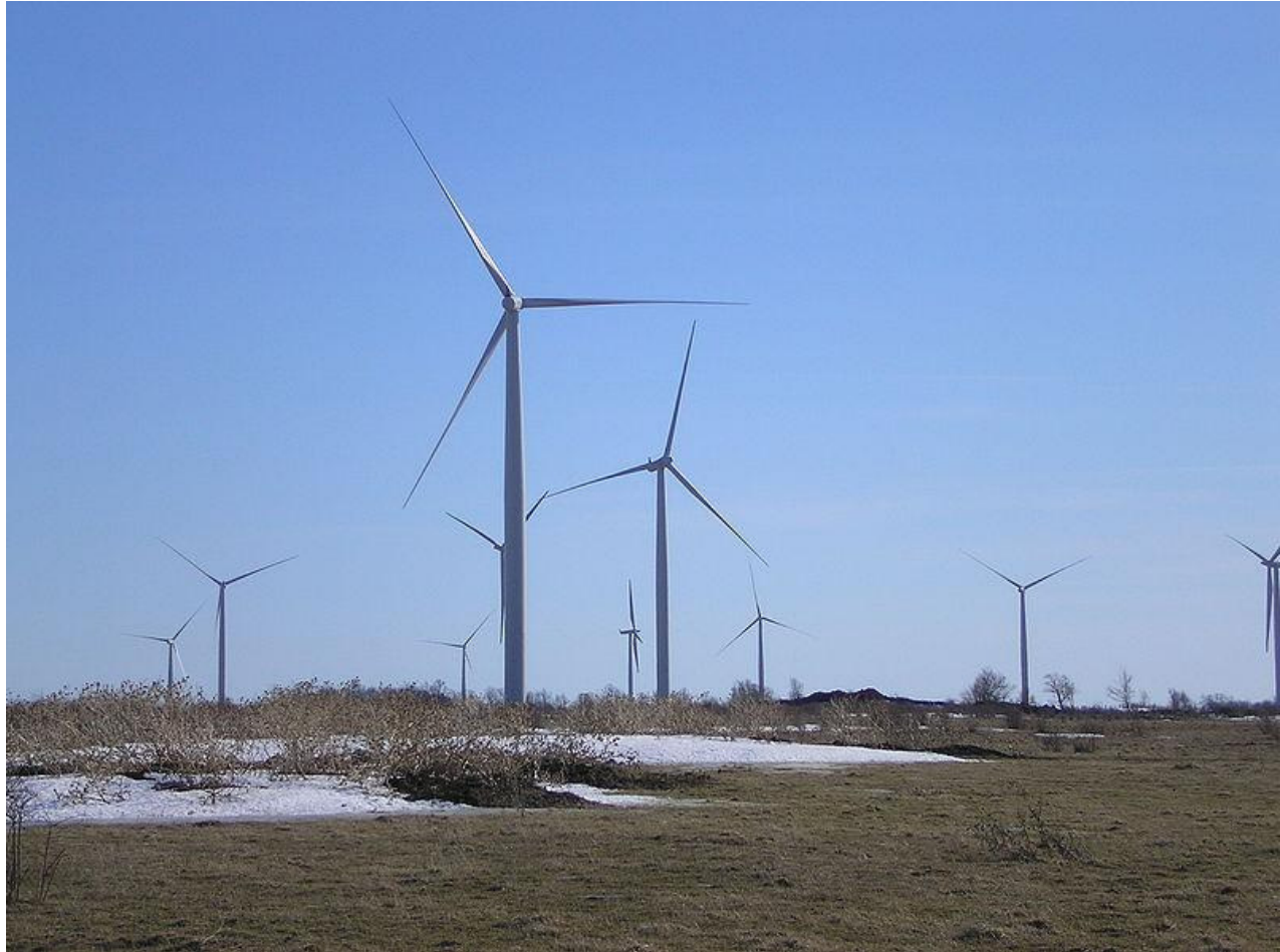
Figure 2-19 Wolfe Island Wind Project in Spring
