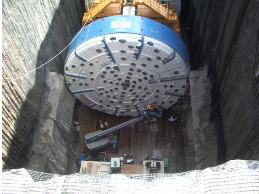
Figure 2-16 Drill Used on Niagara Tunnel Project
