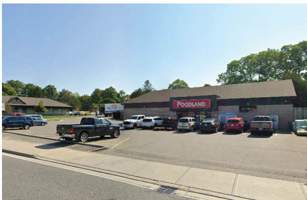
Image 1- View of the Subject Lands Along Alma Street
